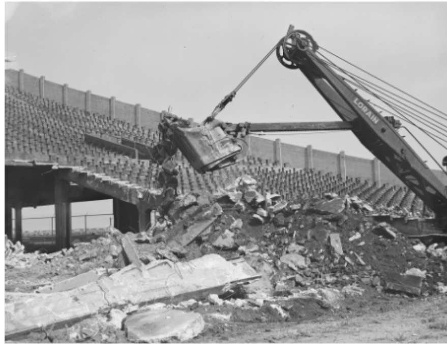
Demolition of Braves Field Grandstand (Leslie Jones, 1955).
