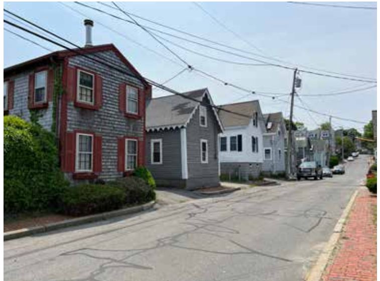
Row of nineteenth-century worker housing, Plymouth, MA.
