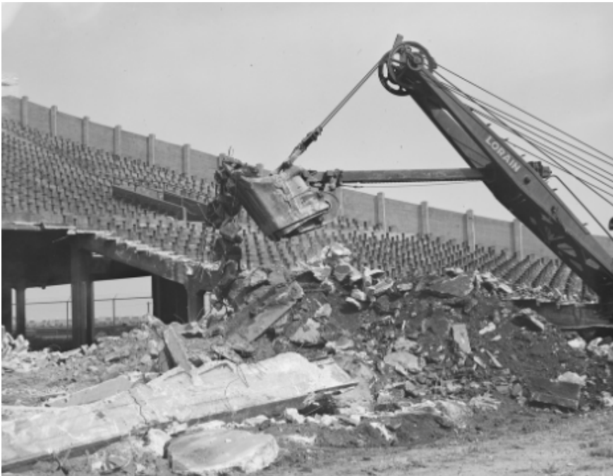
Demolition of Braves Field Grandstand (Leslie Jones, 1955).
