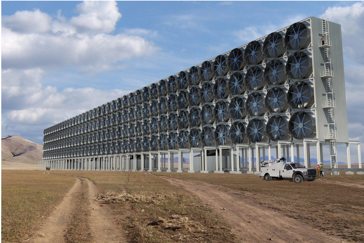
Figure 3: A rendering of Carbon Engineering's industrial-scale air contactor design for direct air capture.
