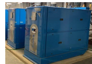
Central hot water boilers
