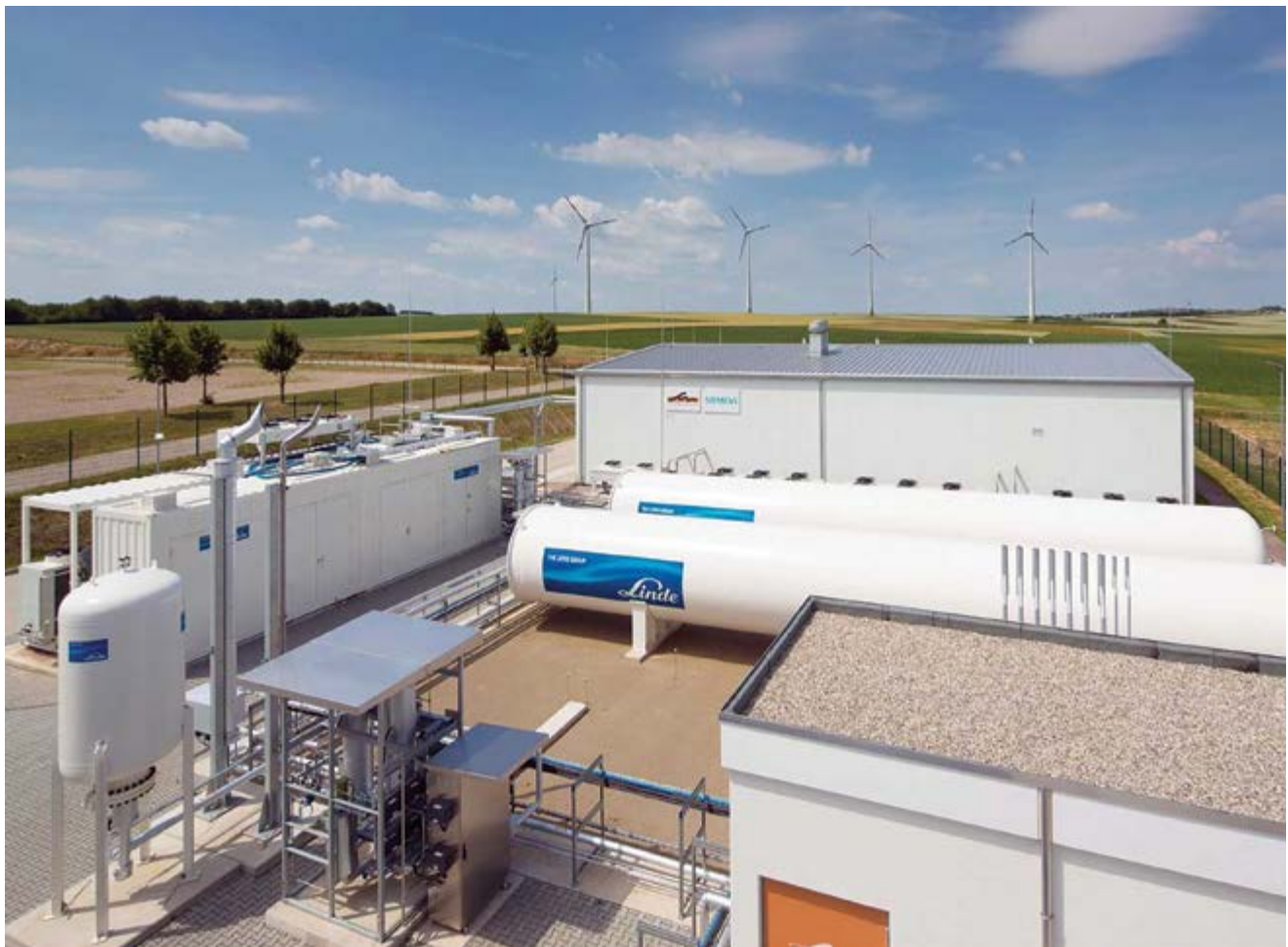
“Energiepark Mainz” located in Mainz, Germany, is connected to an 8 MW wind farm. Three electrolysis units can produce 1000 Nm 3 hydrogen per hour (89.8 kg/h). Photo credit: Stadtwerke Mainz AG
