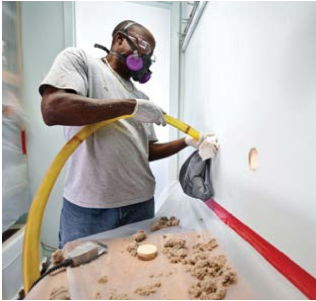
Residential Energy Efficiency. Insulation added to walls reduces heat loss and lowers energy bills. Photo credit: National Renewable Energy Laboratory
