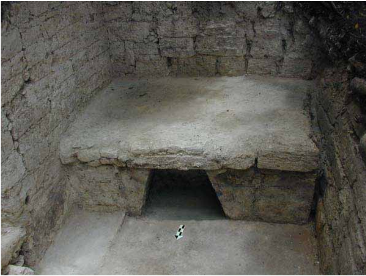
Figure 8. View of Bench 1 in the south corner of the west room (interior room) of Structure 43.
