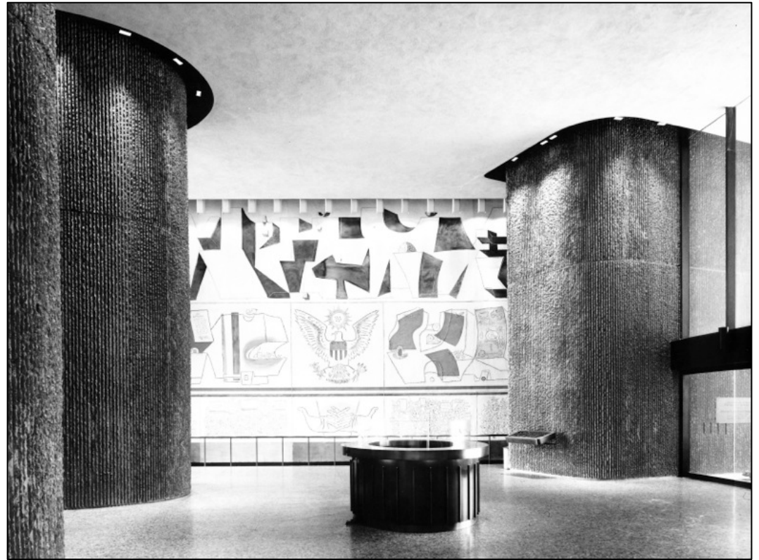
Interior view of the Boston State Service Center, Boston, Massachusetts
