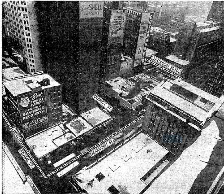
(TRIBUNE Photo) Approximate area to be cleared in Loop for federal building, which will be east of present headquarters. Building will have five story base, with twin towers rising above that level. Plans call for 65 million dollar project. (Story on page 1)
