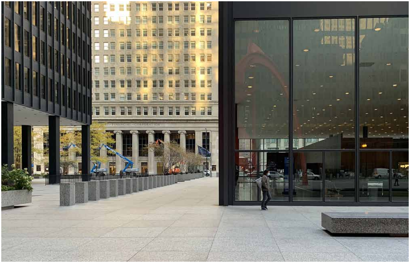
Figure 20 Ludwig Mies van der Rohe, Chicago Federal Center, 1959–74, colonnade of John C. Kluczynski Federal Building at left, aligned with and echoing the colossal order of Graham, Anderson, Probst & White’s Illinois Merchant’s Bank Building, 1924 (photo by Daniel Bluestone).
