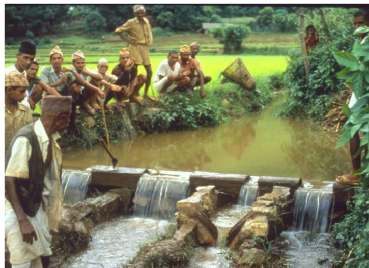
Figure 17: A farmer managed irrigation system proportioning weir in the Palpa district of Nepal
