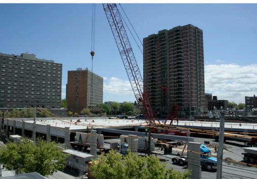
This summer will see completion of the new athletic field's parking structure and an architectural enclosure around the area. Exterior parking will be created for 27 cars or 5 motor coaches. The top of the structure will receive a 240' x 384' synthetic turf playing surface configured for field hockey, lacrosse, and soccer. The open-air field will feature bleacher seating, a brick façade, and enhanced landscaping
