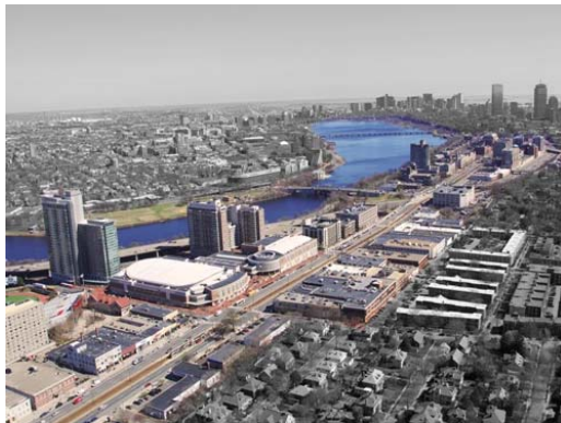
Figure 4-11, Aerial View Looking East
