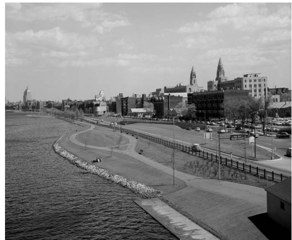
Figure 4-14, Storrow Drive After Construction
