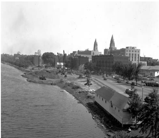
Figure 4-13, Construction of Storrow Drive
