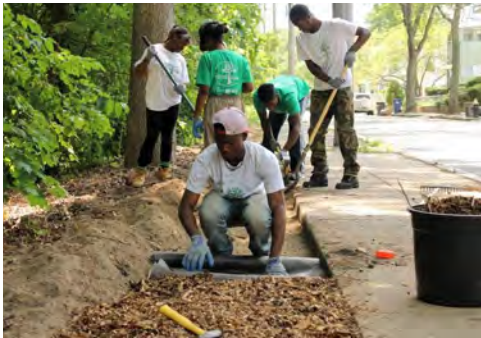
Boston Green Team Southwest Corridor CDC
