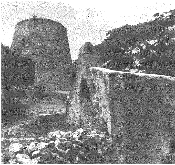
Windmill towers are perhaps the most easily recognizable structures of sugar plantations. Large wooden sails, powered by the wind, would drive rollers used to crush the juice from the sugar cane. The bake oven in the foreground was used for baking most of the bread consumed by the estate's slave population. These are located at Annaberg Plantation, a late 18th-century sugar plantation now owned and maintained by the National Park Service.
