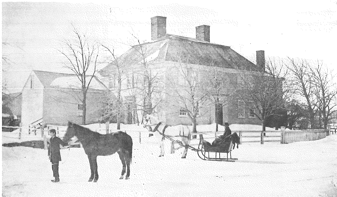
In this earliest-known photograph of the Golden Ball Tavern (1868), the East Ell can be seen attached to the left of the main house.
