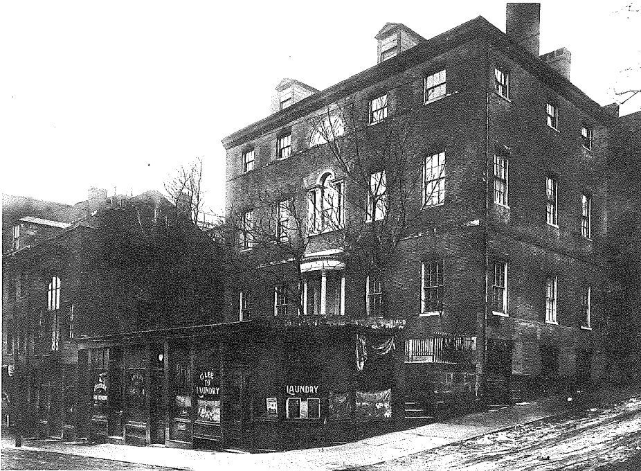
The Otis House in 1922 soon after the Federal style façade was restored by SPNEA. Photograph from SPNEA archives.
