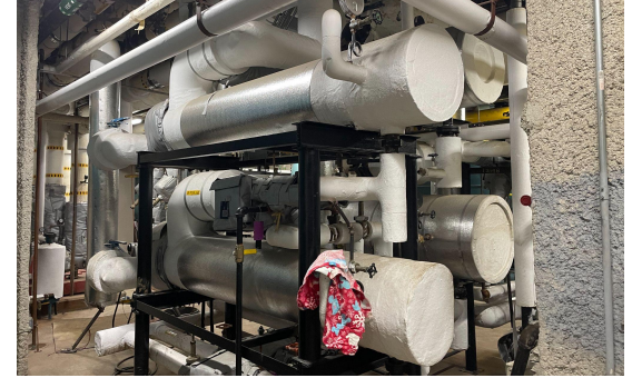
StuVi-1 Heat Exchanger
