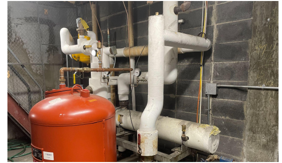
Claflin Hall Heat Exchanger
