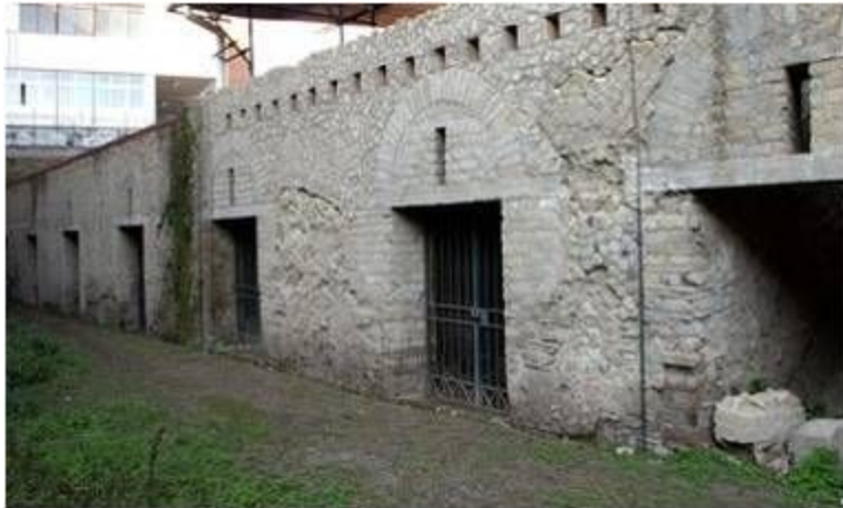
Figure 2. Exterior of sea-facing storage rooms, including room 10, Oplontis B. (Photo: copyright the Ministero dei Beni Culturali e il Parco Archeologico di Pompei).
