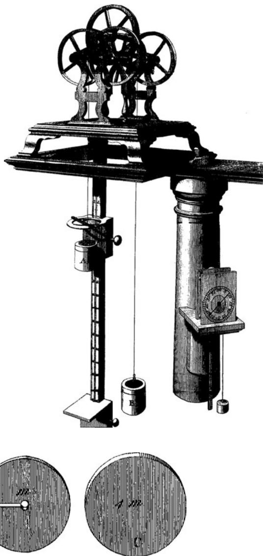
**Fig. 17** Three pieces used to vary the weight of the boxes (Atwood 1784, fig. 81, 80, 79). The symbol “m” on the pieces does not represent mass but rather weight,  $m = \frac{1}{4}$  oz
