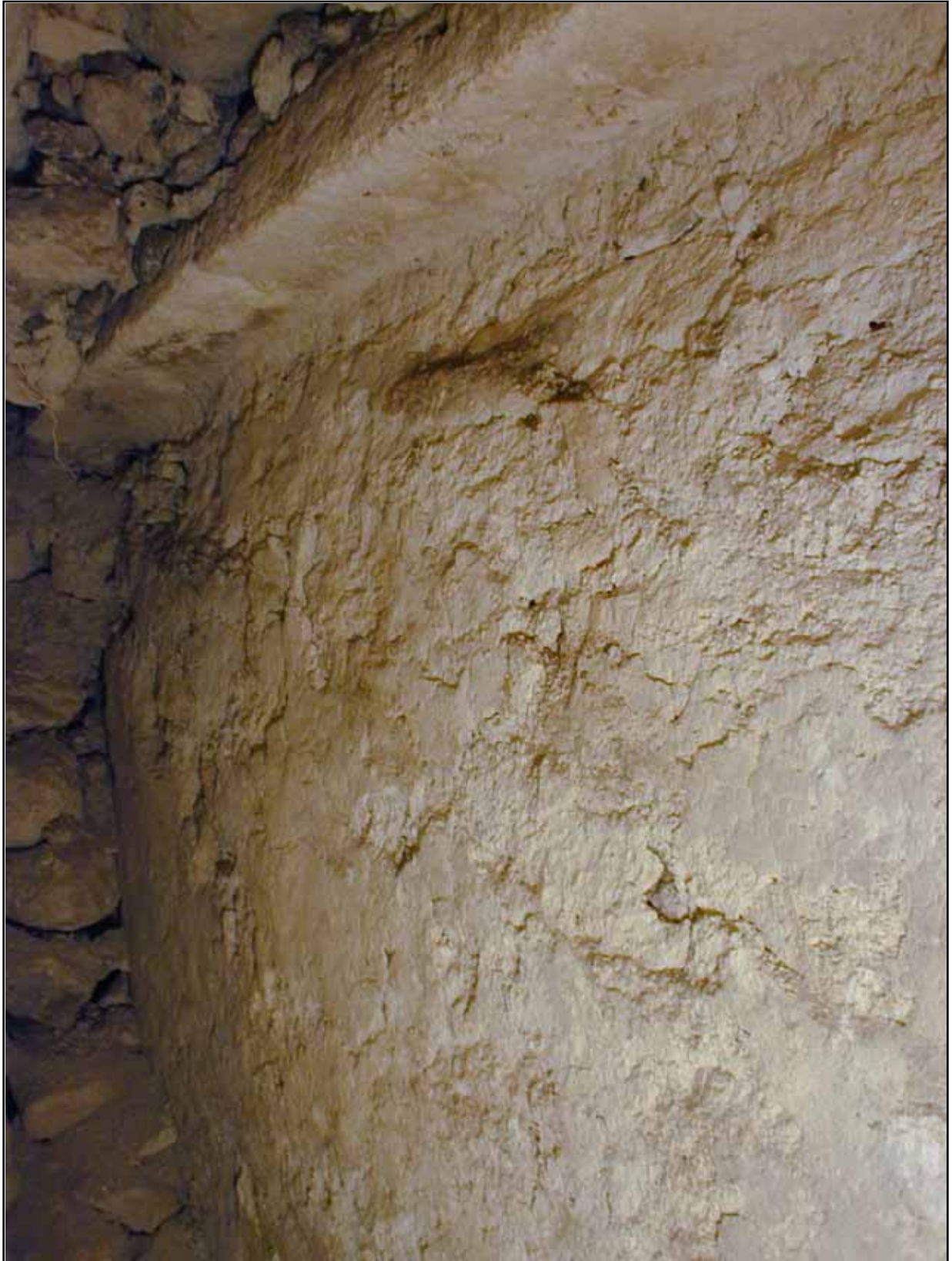
Figure 13 Southern wall of Structure 1 sub 3 with cornice
