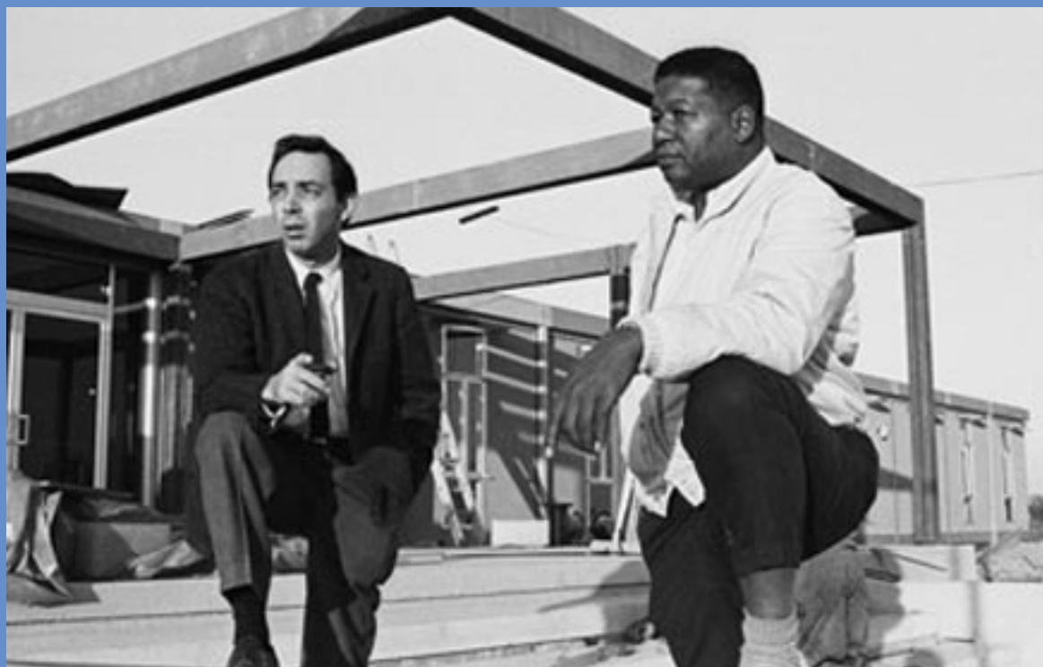
Dr. H. Jack Geiger and Dr. John W. Hatch during construction on the Delta Health Center, 1968 Photograph by Daniel Bernstein
