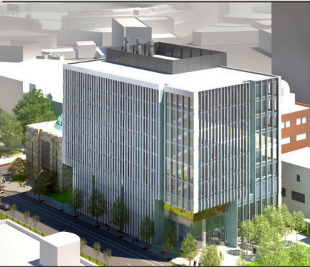
The Center for Integrated Life Sciences and Engineering Completed Spring 2017
