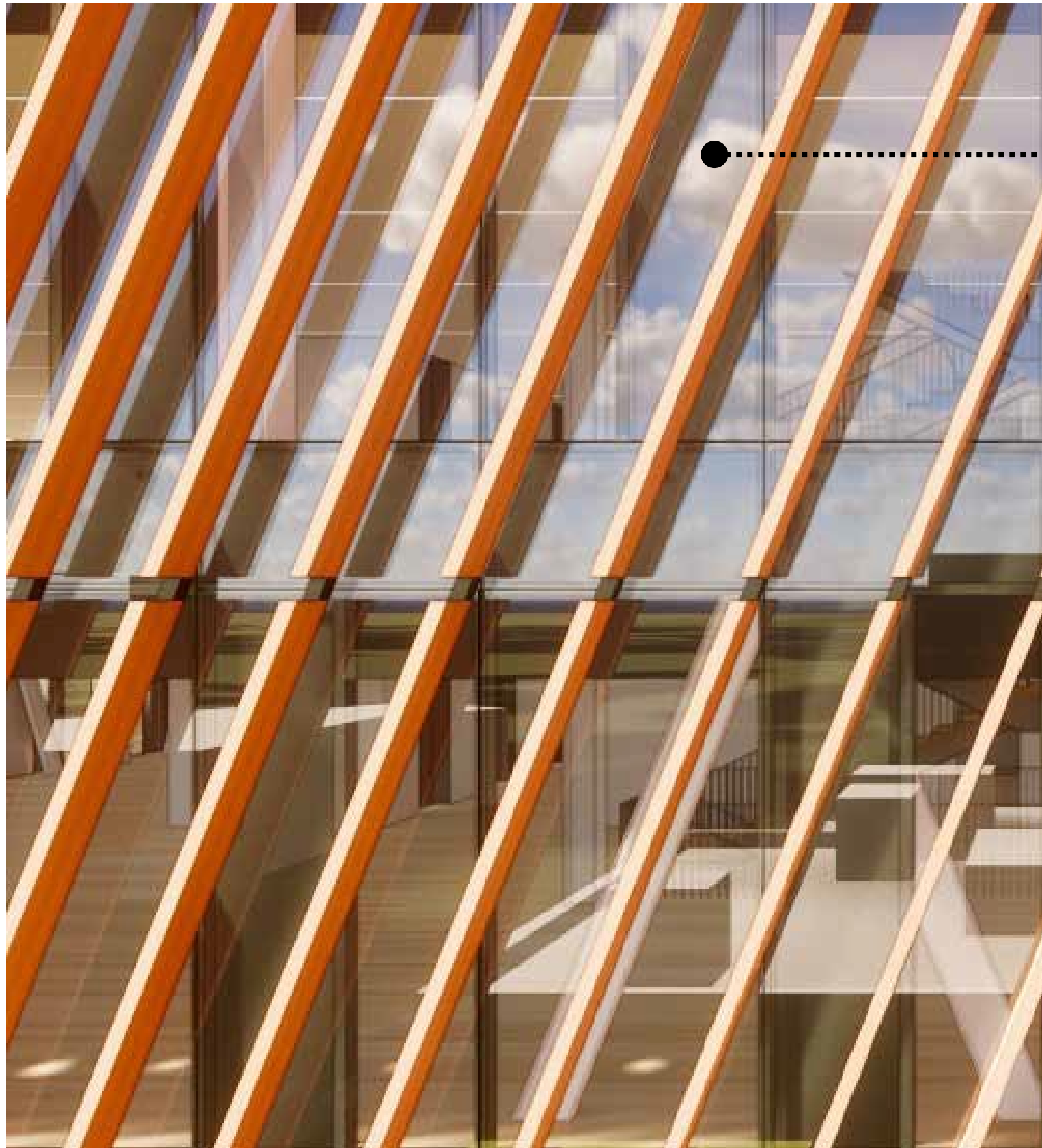
Diagonal Louver Facade Design
