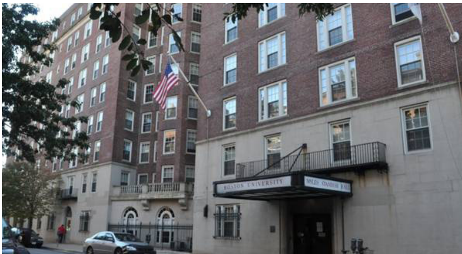
Photograph 5: Existing Myles Standish Hall as seen looking east from Bay State Road
