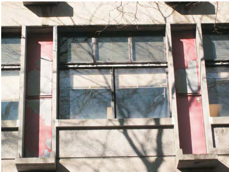
Typical Window Treatments on Tower
