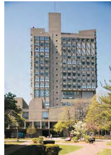
View of Pappas Library Building and Tower Looking West
