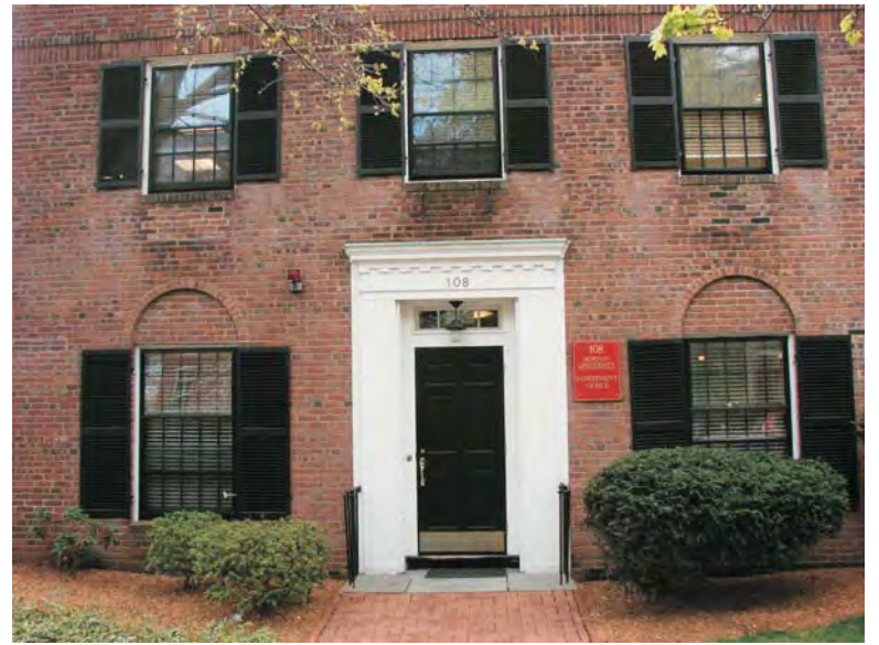
View of the Building Facade
