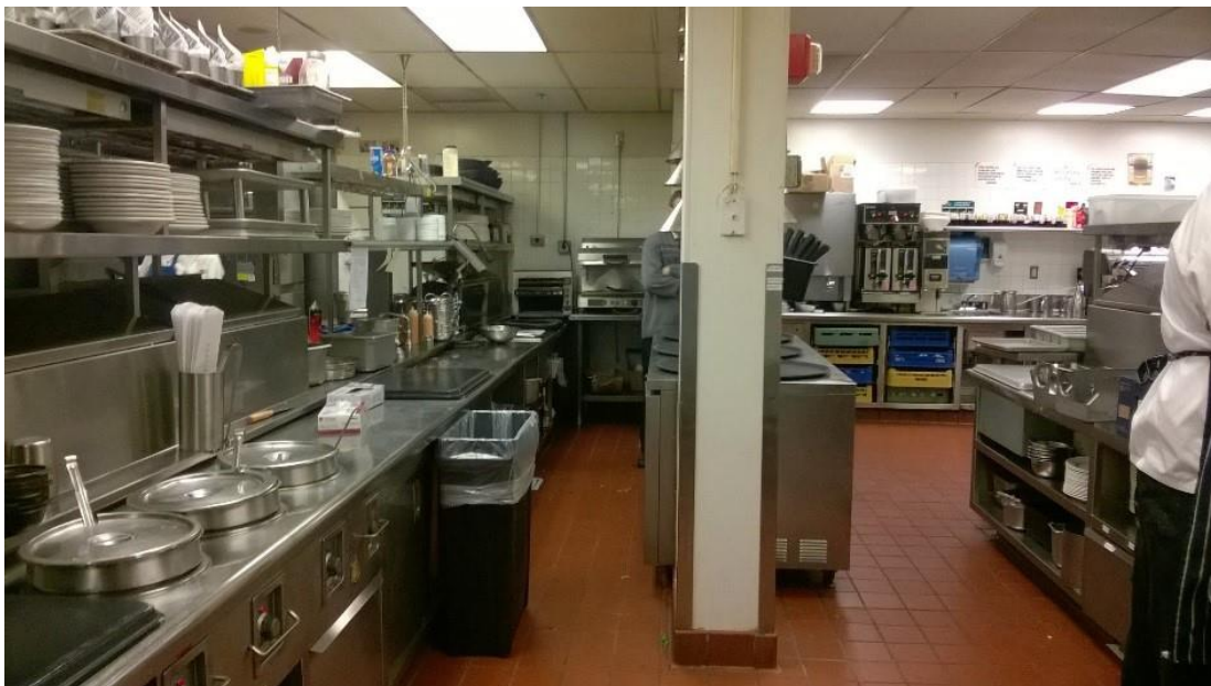
Brasserie Joe – The island pass is located in the middle of the kitchen (Hidden by pole).
