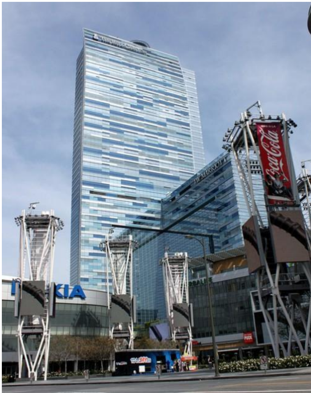
1 Behind Los Angeles' Staples Center sits the dual-branded JW Marriott and towering Ritz-Carlton (Photo by Prayitno)
