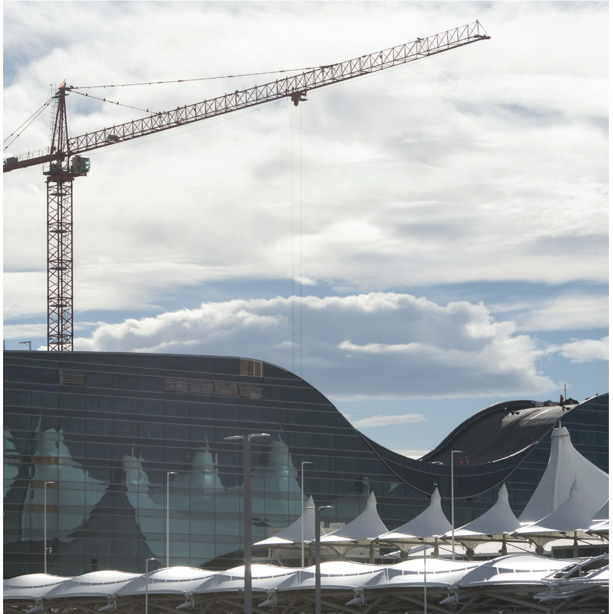
Right, Construction of the Westin Hotel at the Denver International Airport
