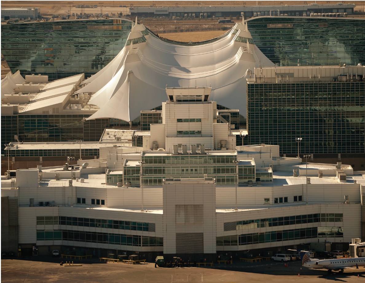
Left, The completed Westin Hotel at the Denver International Airport
