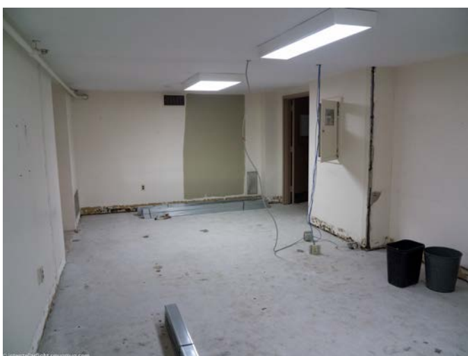
Renovation of the Astronomy main office. Image shows the space that was converted into a small conference room and the administrator's office.
