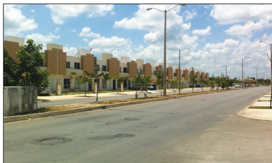
A new Infonavit-era housing development in Cancún. Homes in so-called social interest housing projects such as this one are built with shared walls in order to increase density and lower cost. Photo: G. Hartman
